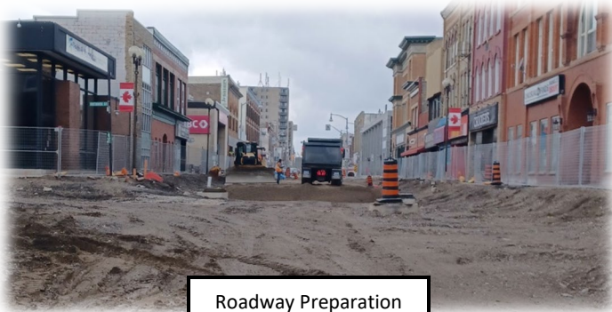
Roadway Preparation Granular being placed
