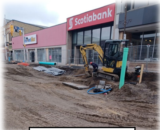
Electrical duct installation
